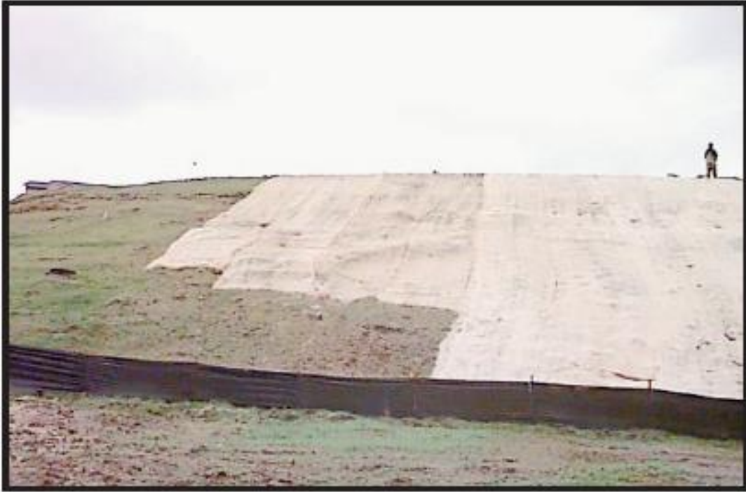
Plate 3 – Coconut matting and silt fence (Source: CIRIA, 2006 10 )
